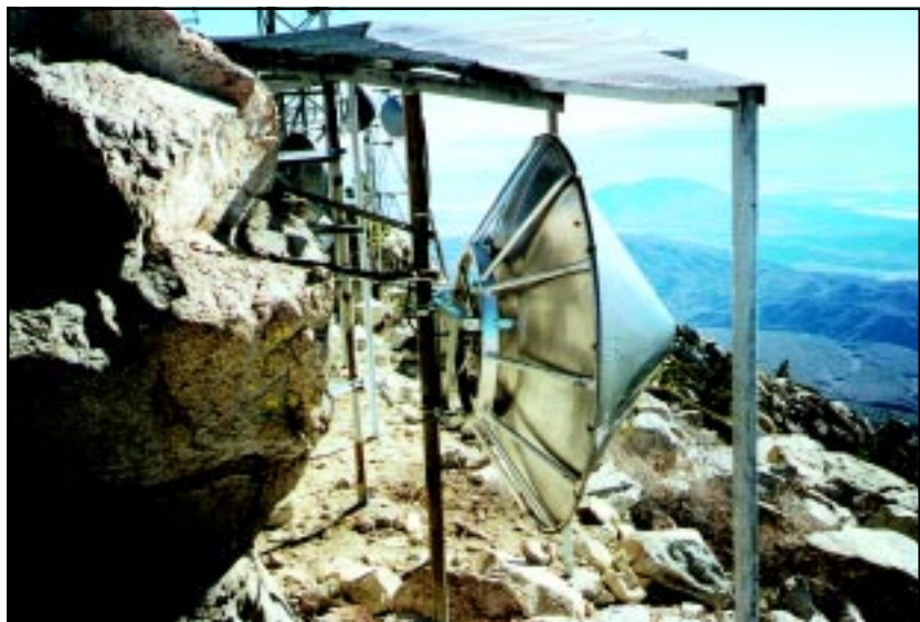
Real-time data are collected at Toro Peak in southern California from remote seismic stations using radio telemetry for PASCAL Broadband Array tests and the ANZA Broadband Seismic Network operations. The data are sent through the Internet using the microwave link shown in the photo. [photo: G. Offield]
